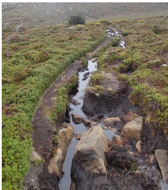
Photo 2. Eroded and braided alpine section of the Mt Oakleigh side track.
