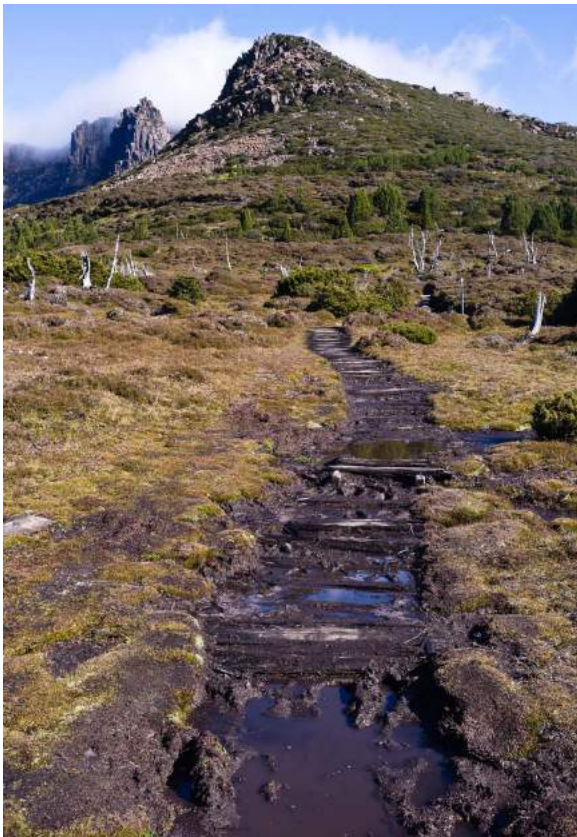
Photo 4. Widening trampled corridor as walkers avoid derelict cordwood. Hardwood logs were laid to provide a hard surface in many muddy peat areas along the Overland Track during the 1980s. Many have now rotted and become a derelict, uneven tread surface that requires replacement.
