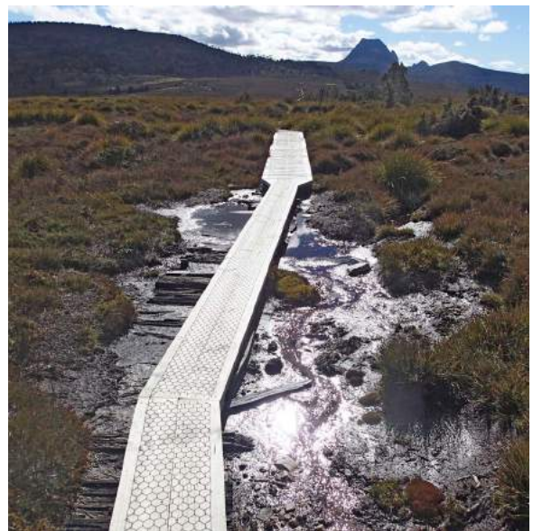
Photo 6. “Planking” is a modern track hardening technique that is relatively efficient and cheap to lay. By 2015 planking had been used to harden 13.3 km of the Overland Track.
