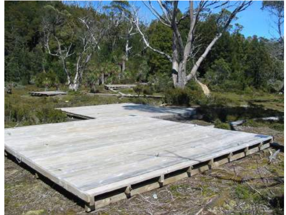
Photo 5. Timber camping platform at Windermere, typical of those installed at most major overnight nodes on the Overland Track since 2001.
