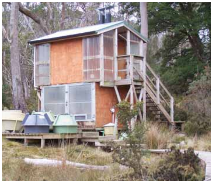
The new toilet for the new Pelion Hut, also on the edge of the Pelion Plains [Photo: A. McConnell]
