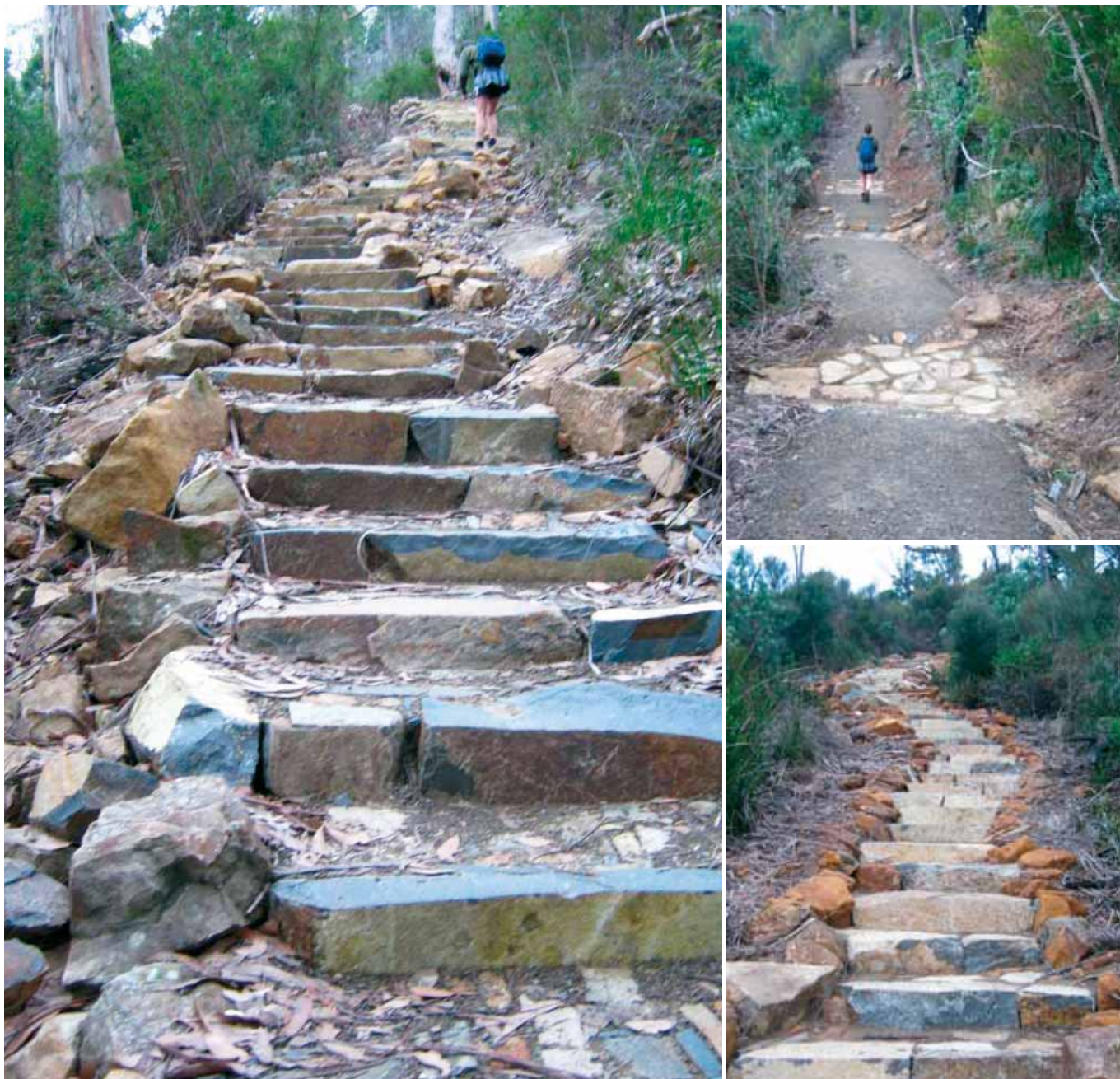
Recently upgraded Fortescue Bay – Cape Hauy Track (Jul 2012, photo – A. McConnell)
